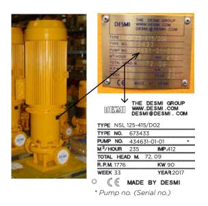
Pump no. (serial no.) is punched into the flange of the pressure side.
