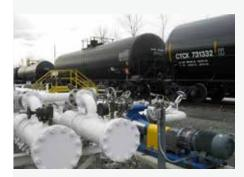
Sound Refining receives heavy oil and asphalt by rail. Two specially selected RO-TAN® pumps handle these products where extreme suction and discharge capability is appreciated. As described, the ROTAN®'s pull and push a ton.
