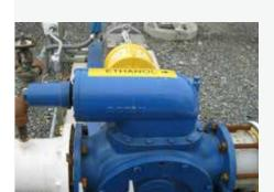
A similar ROTAN<sup>®</sup> model HD201 delivers Ethanol to distant storage. The delivery rate exceeds expectations. Tom Beck comments, "despite incredible discharge pressures, they have yet to see even a drip leak from the mechanically sealed ROTAN<sup>®</sup> pump".
