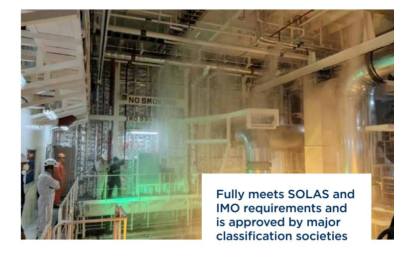
The FineFog™ local application system lets you protect high-risk objects in accordance with SOLAS requirements without having to shut down the engine and evacuate personnel. Its fire suppression or extinguishing function is based on water mist nozzles complemented by DESMI design for easy and safe operation during the entire lifetime of the product.
