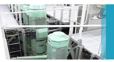
Many vessels are equipped with a general service pump which can be used for more applications such as e.g. bilge, ballast or fire.
