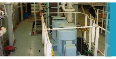
The NSL pump is the most obvious choise for this application. It is vertical to save deck space, it is reliable, and it can handle the high pressure required due to the special impeller design which takes a lot of the pressure away from the shaft seal. The NSL pump is also designed to handle the pressure of the big electric motor which is often required to operate a fire pump.
