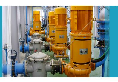
Most vessels have one or more boilers onboard for different applications such as exhaust gas or oil fired boilers. If the boiler is filled with water it is recessary to re-fill it with water when steam is leaving the boiler. For this purpose a boiler feed water pump is needed
