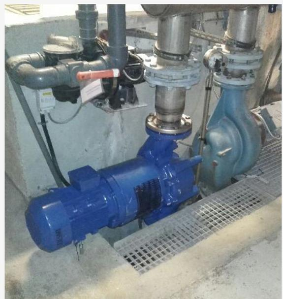
672674 - NSL125-215/D02-p DESMI Pump installed horizontally
