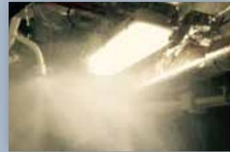
DESMI Water Sprinkler System is a conventional sprinkler system designed as a so-called wet pipe system. A wet pipe sprinkler system is fixed fire protection using piping filled with pressurized water supplied from a dependable source.
