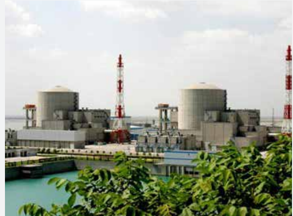
Tianwan Nuclear Power Station in Jiangsu province.
