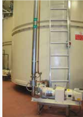
DESMI ROTAN® pump pumping chocolate from one of the big chocolate tanks
