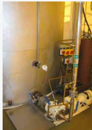
DESMI ROTAN® pump pumping chocolate at the Kinnerton factory.
