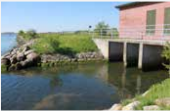
Rain water drained off from the pumping station into Odense Fiord
