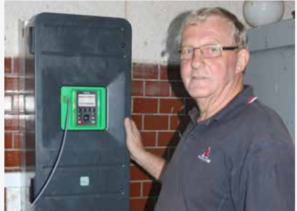
Fritz Hansen, chairman of the pump guild, in front of the frequency converter installed by DESMI in connection with rebuilding and installation of a pump at the pumping station in Lumby
