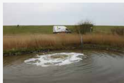
A lake of 260 ha is situated on the other side of the flood defence at the Wadden Sea. At the end of the lake sea water is pumped into the lake from the Wadden Sea.
