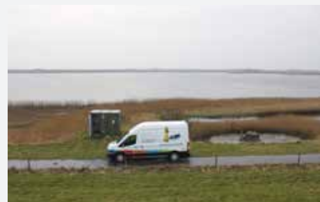
View from the flood defence over the lake, where the pumping station and frequency converters are located.
