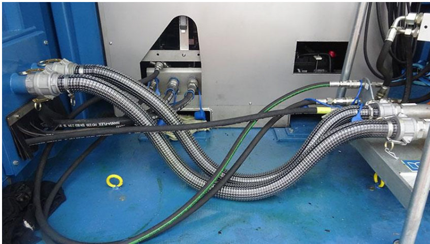
Connect both Air hoses from the Air Blower to the Container bulkhead.
