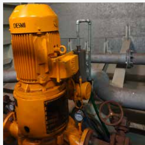
Technical information on the NSL Centrifugal pumps : 150 m 3 /h x 1,52 bar x 1470 rpm Casing Material: Bronze (RG5) CC491K NiAlBz (CC333) impeller Electrical-Driven Priming Pump 1/5 bar manometer Motor: IEC MOTOR 3D3 160 M-4 11/13,2KW / 3 x 400V, 50 Hz / IE3
