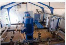
The three NSL pumps and frequency converters installed in Aabenraa.
